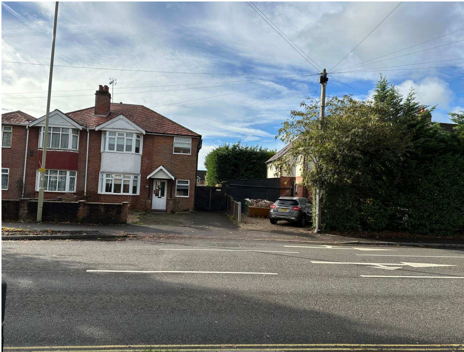
(09) Photo looking South across Leigh Road at the front elevation of No.189 Leigh Road in context with No.191's mature planted shrub boundary, highlighting the form, material composition and extent of visual gap between the two properties.
