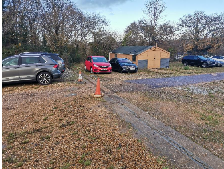
Figure 5: Photo of existing drainage
