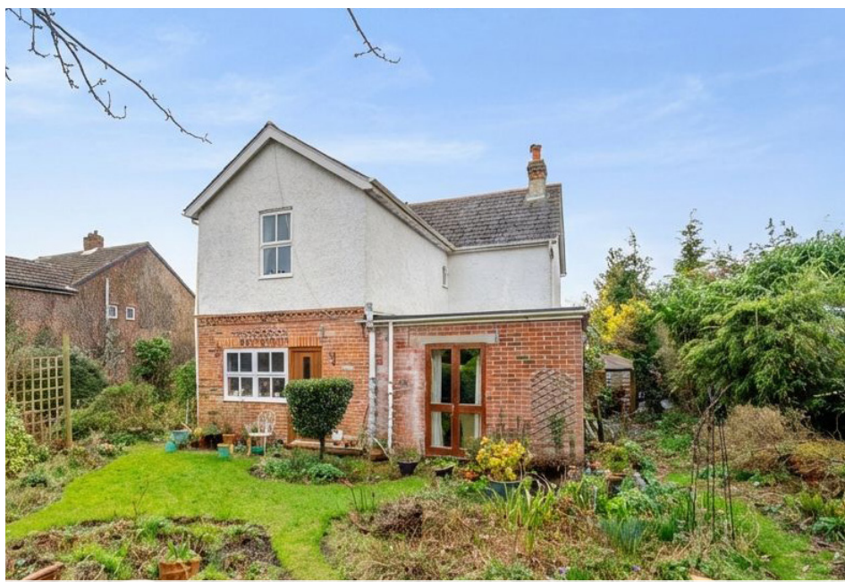
Figure 17: Existing Rear View Photograph manipulated with ai to remove the tree hiding the single story flat roof extension. Original photograph to the right.
