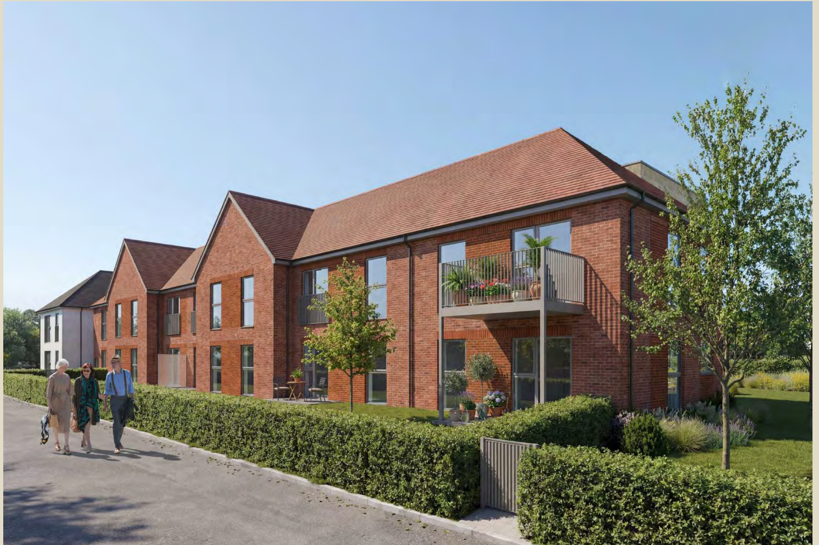
View from northwest corner
