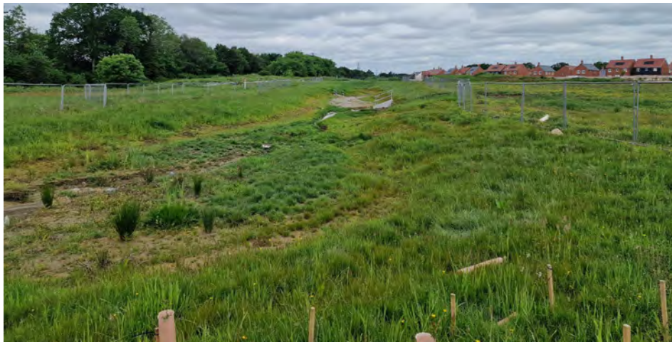
Figure 34. View of Pond 2, dried up at time of inspection (taken May 2024).
