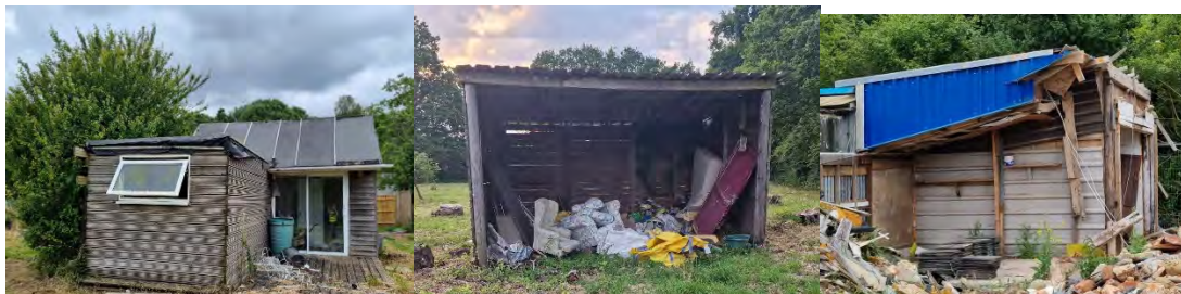
Figure 3. Examples of Buildings - Developed land, sealed surface present on-site (taken January 2026).
