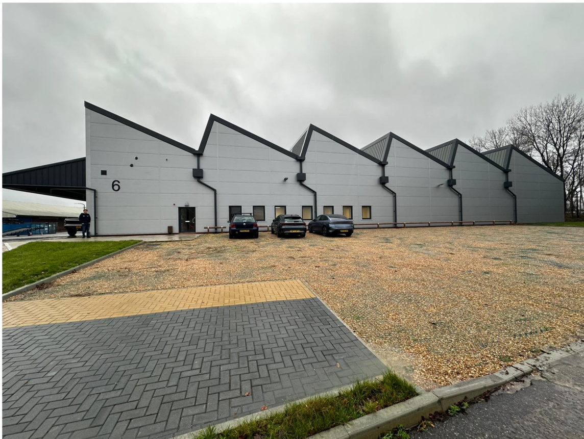
North west elevation of unit 6
