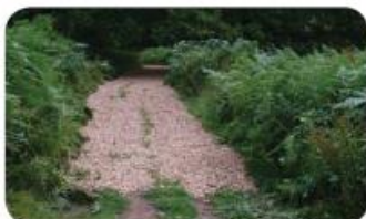
Step 1: Prepare Surface
