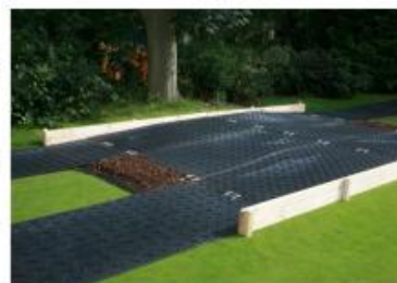
Ground-Guard trackways should have additional cushioning installed where they pass near to trees.
