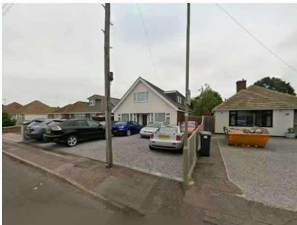
The side flat-roofed dormer at no.26 Monks Brook Close.
