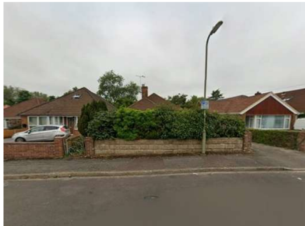
The application site viewed from the east, on Monks Brook Close.
