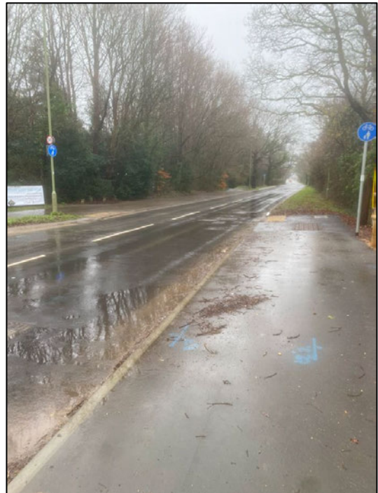
Photograph 2: Existing Footway Conditions
