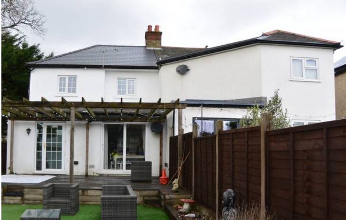
Fig.3 Existing view on the back of the property showing chamfer to Hawthorns
