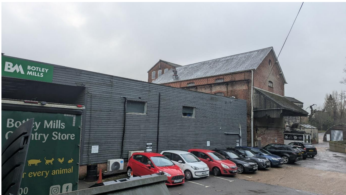
Limited view of provender mill building viewed from the east
