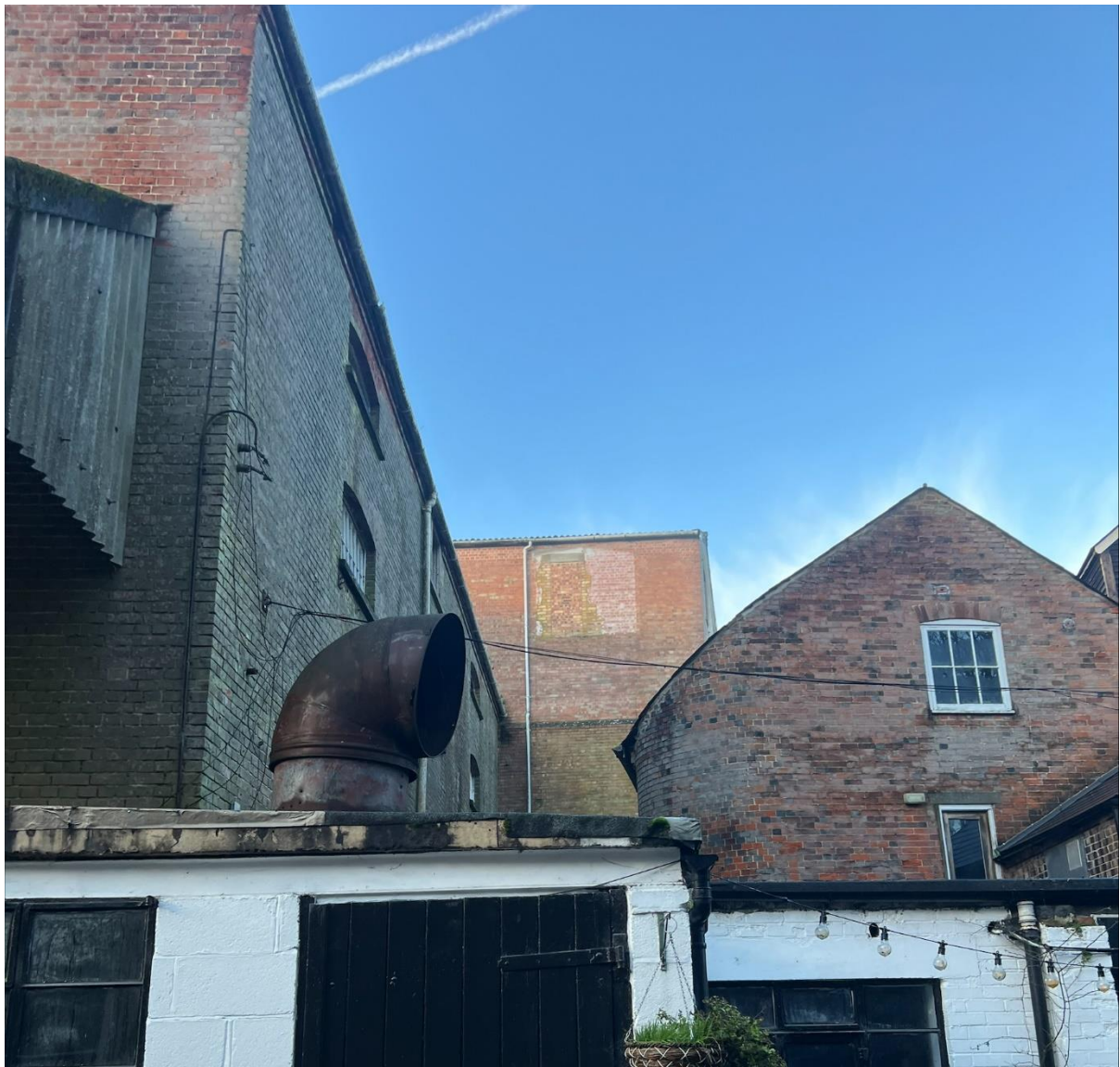
View of provender mill between adjacent buildings to the east
