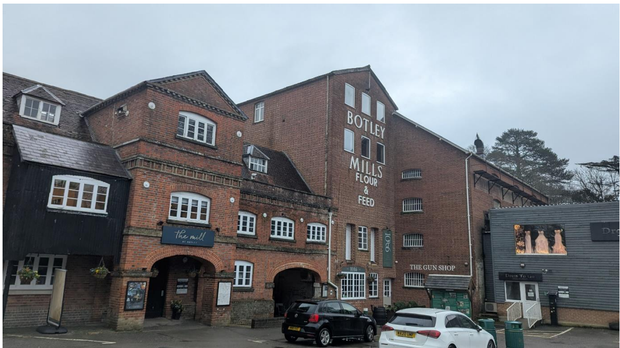
Photo demonstrating that face of roof to provender mill is not visible within the site
