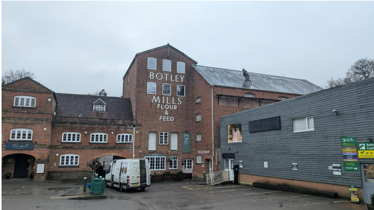
Front elevation of building; the provender mill building is in the centre
