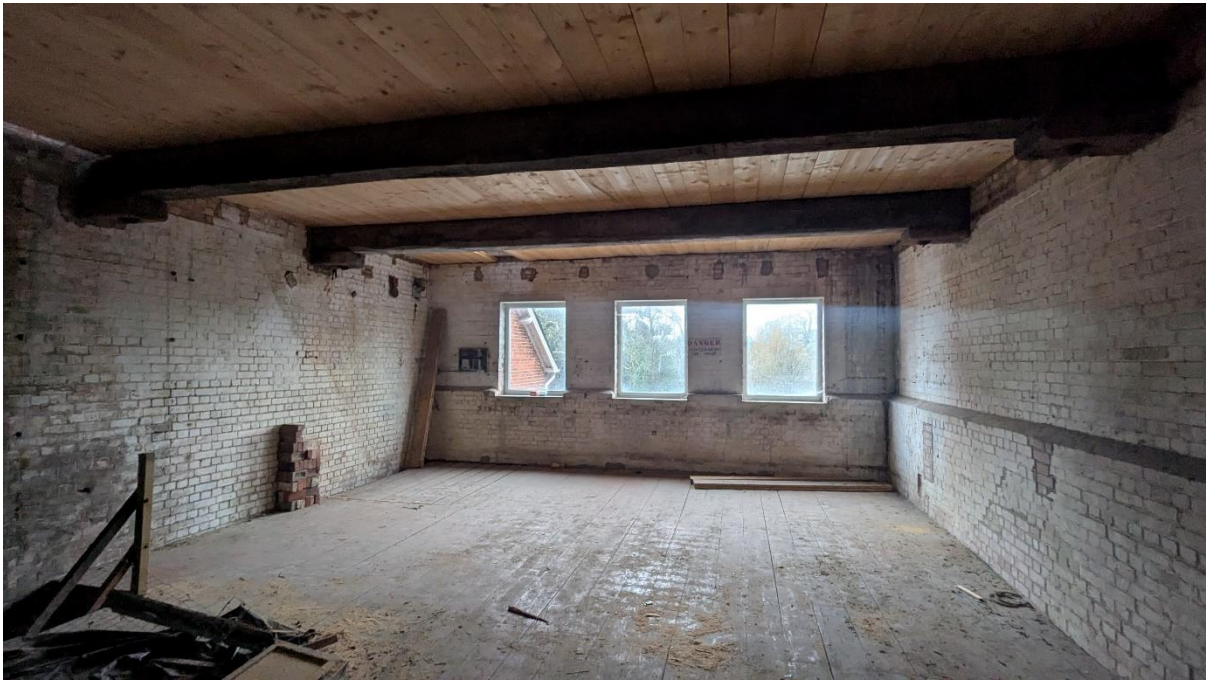
Typical interior view of the third floor level
