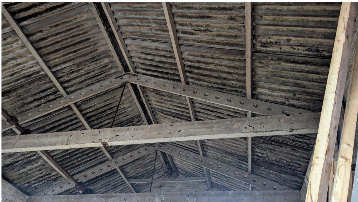
Internal view of roof showing timber trusses and purlins
