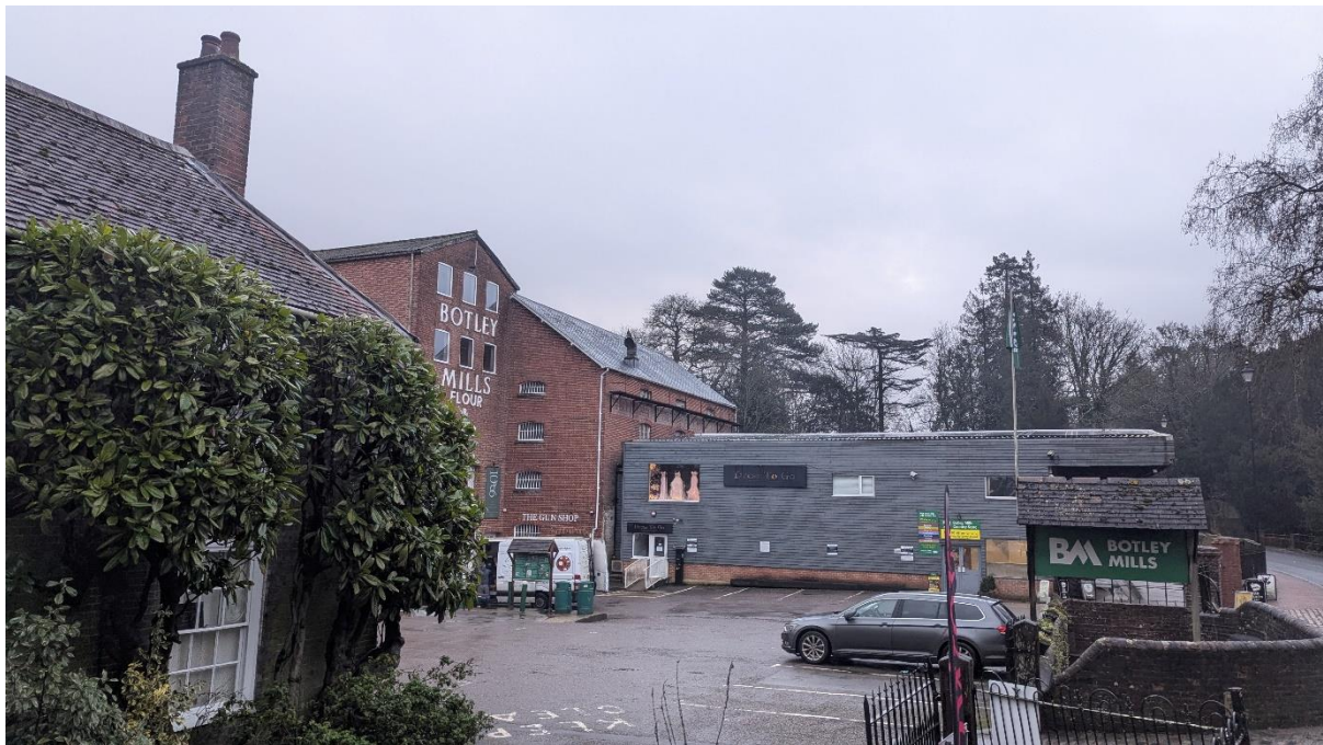
View of site from Mill Hill, showing that surface of the roof is only just visible
