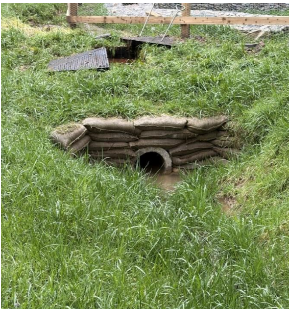
Figure 1.8: SuDS Outfall headwall
