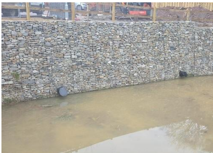
Figure 1.3: Flap Valves installed on the outlets to the SuDS Feature
