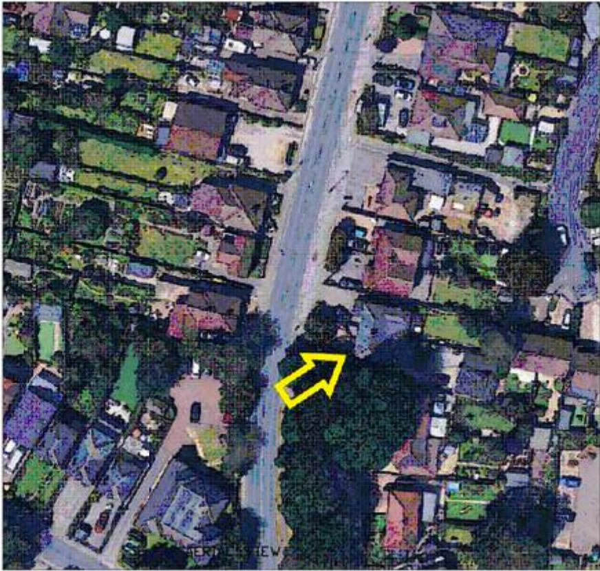
AERIAL VIEW ON SITE
