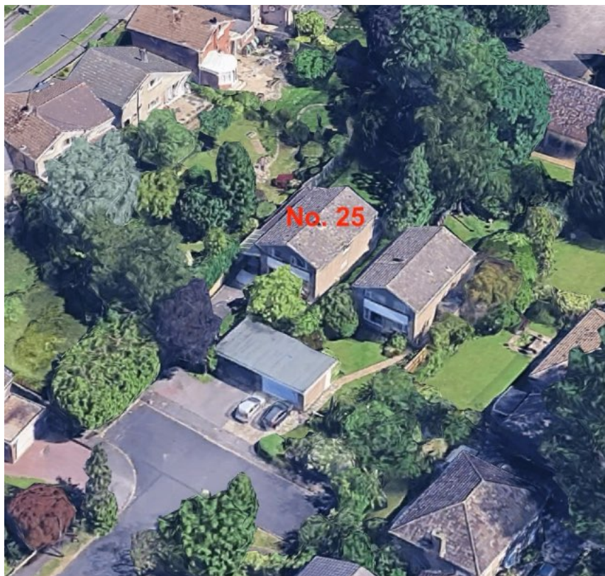
Figure 3 Aerial View - Google Maps 3D Image
