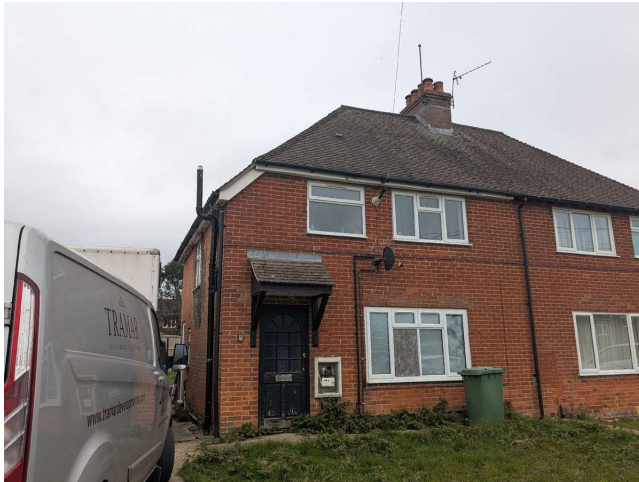
Photo 5: B1 - southern elevation
