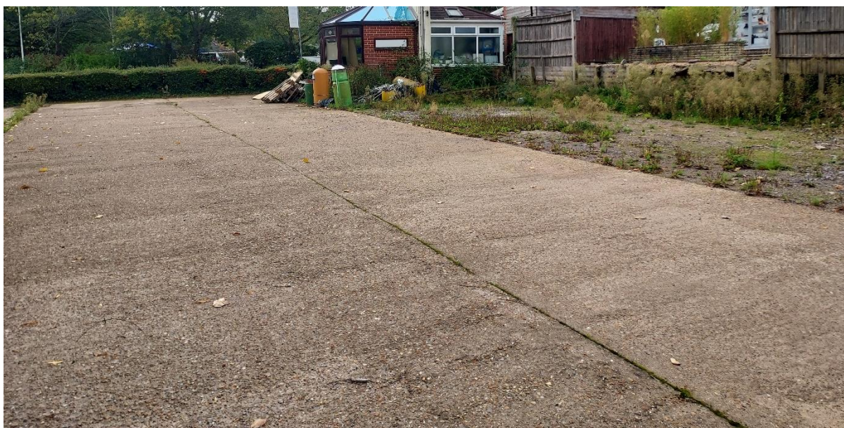
Photo 3: Area of concrete slab with some vegetation growing at the edge of the site to the rear
