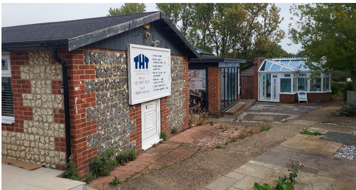
Photo 4: The main building with a ridged fake tile roof and the conservatory building to the rear
