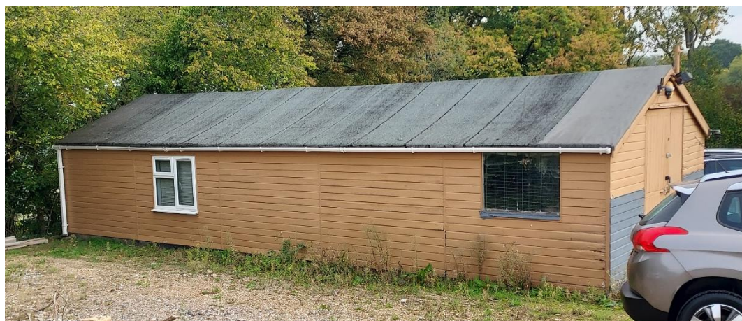
Photo 6: A shed used on site
