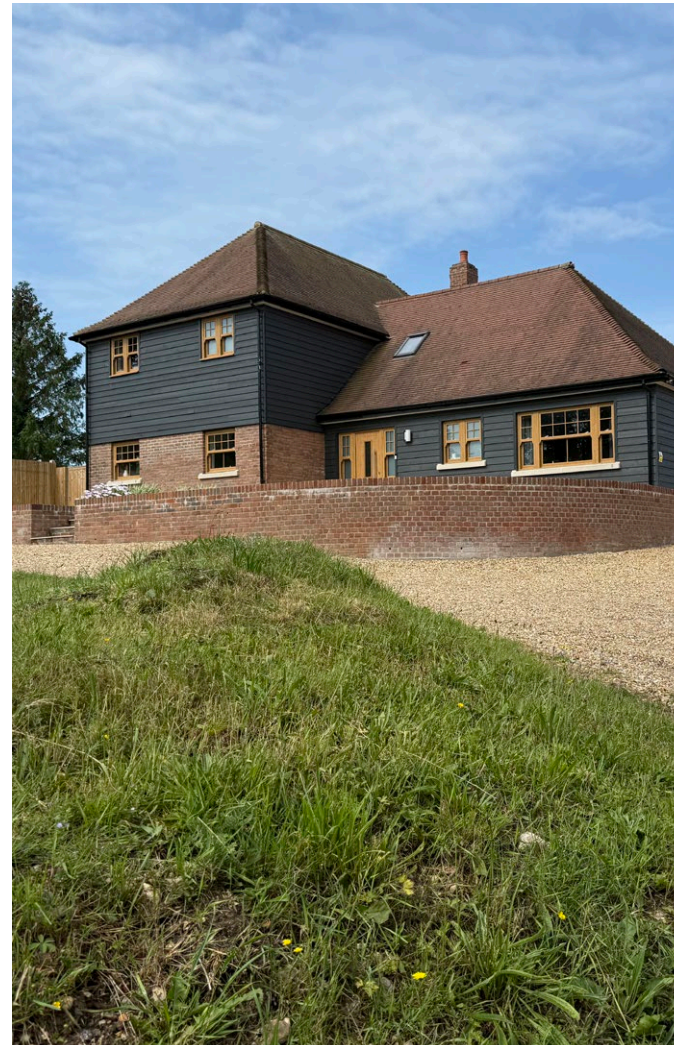
Fig 4. Recently constructed dwelling with garden that projects into the north-east corner of the Site opposite Maddoxford Farm
