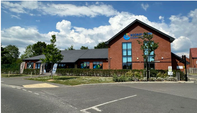
Fig 11. Boorley Green Community Centre
