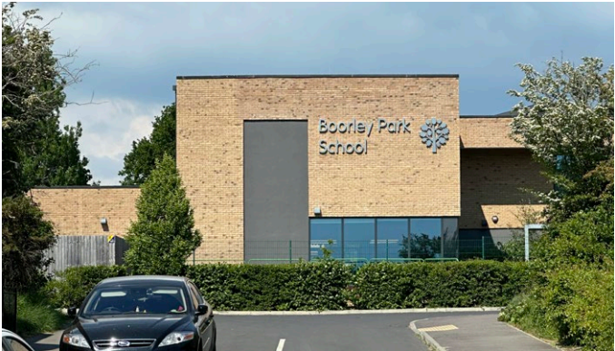
Fig 12. Boorley Park School
