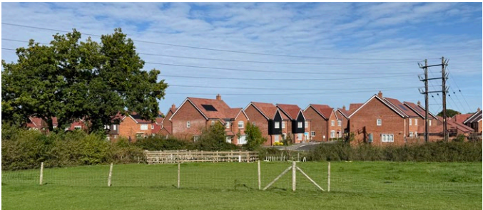
Fig 19. Existing overhead electricity lines in north-west corner of the Site to be retained and developed around
