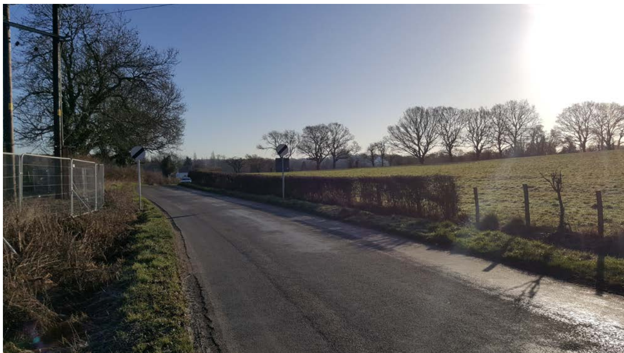
Plate 11 View of overhead power and gas main crossing point on Maddoxford Lane
