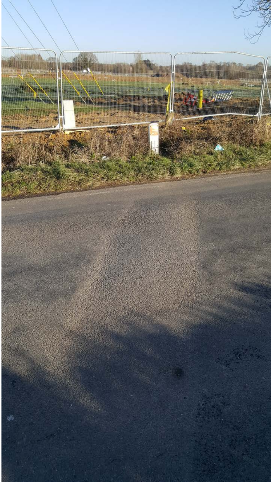
Plate 18 View of Scar in Maddoxford Lane and gas pipeline marker scar traces back across the western field
