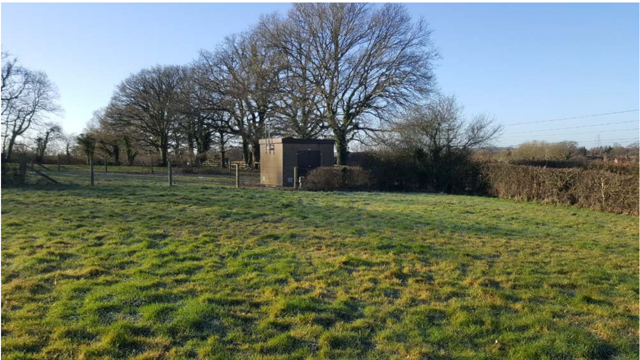
Plate 4 View of Gas Valve Compound immediately to south of western field
