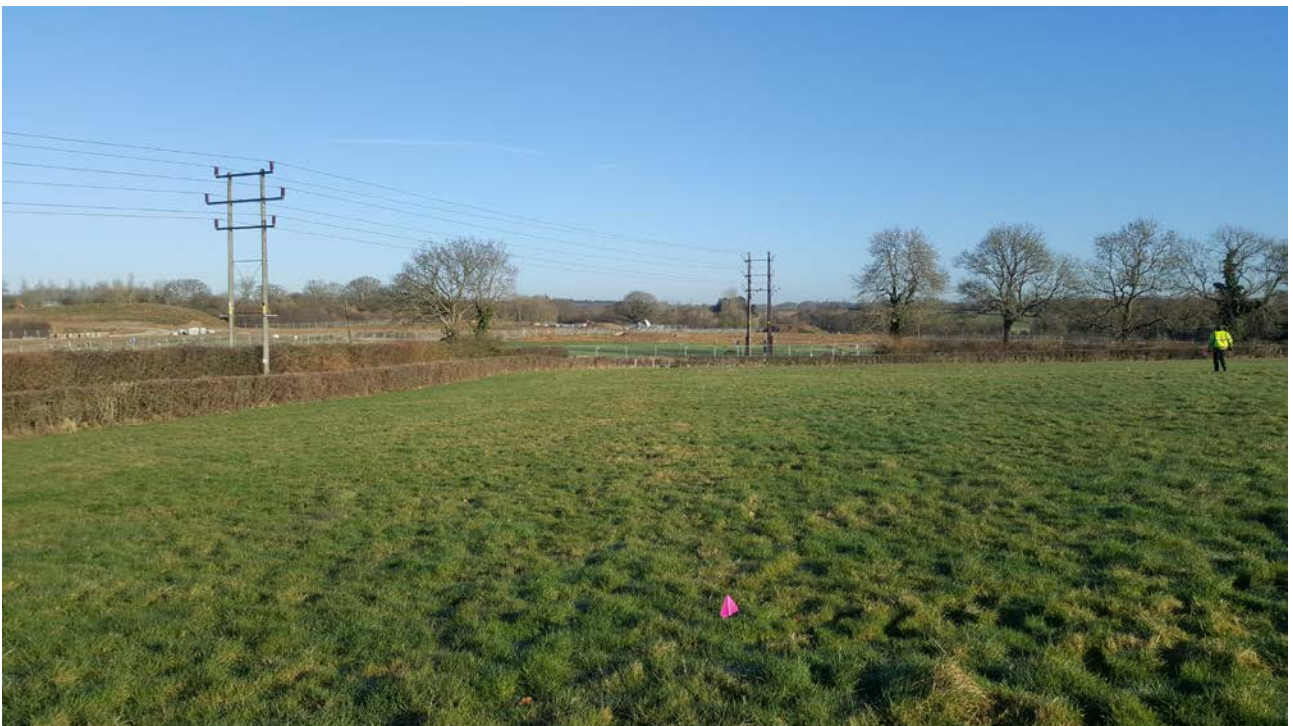
Plate 10 View of marker flags along gas pipeline route through western field
