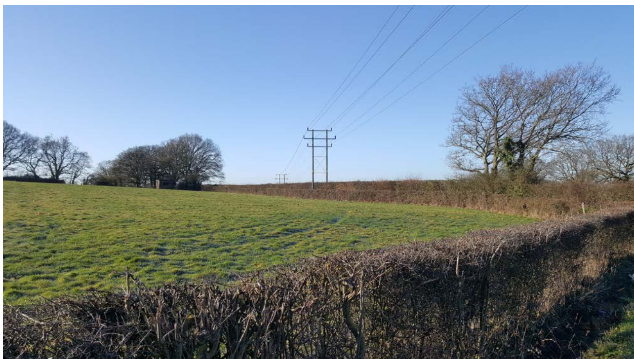
Plate 14 View of overhead power lines in NW corner of western field
