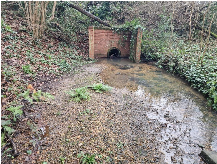
Figure 11. Spear Pond gully, found within 250m of the site boundary (Taken February 2026).
