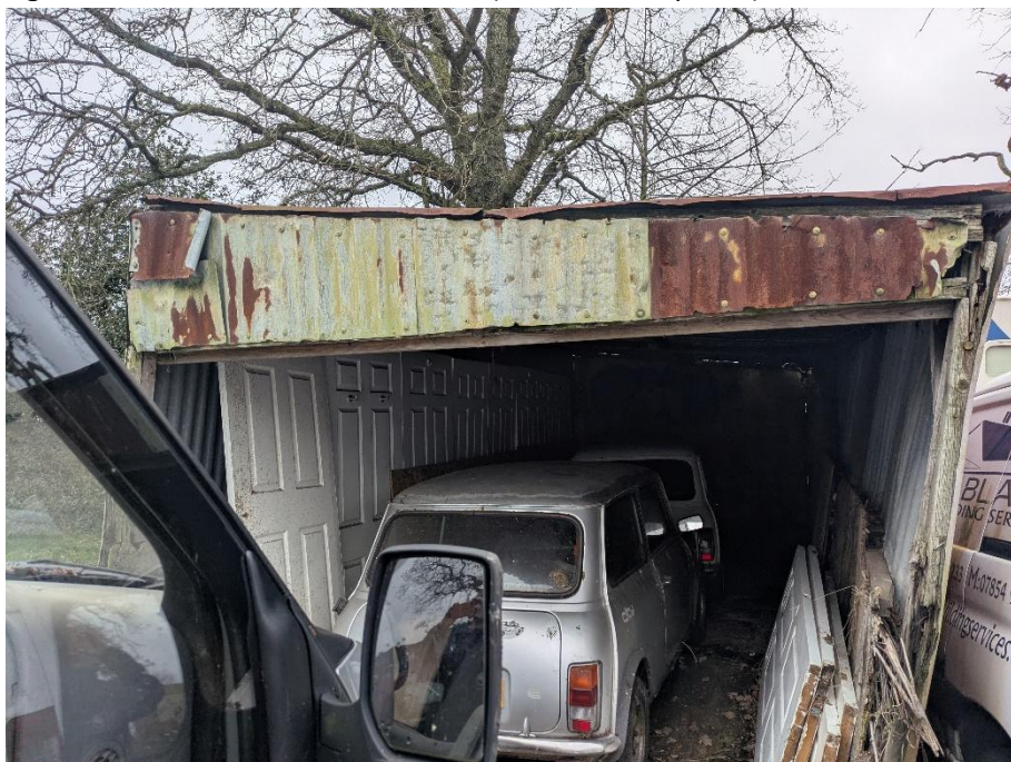
Figure 10. Wooden framed shed on site (Taken February 2026).
