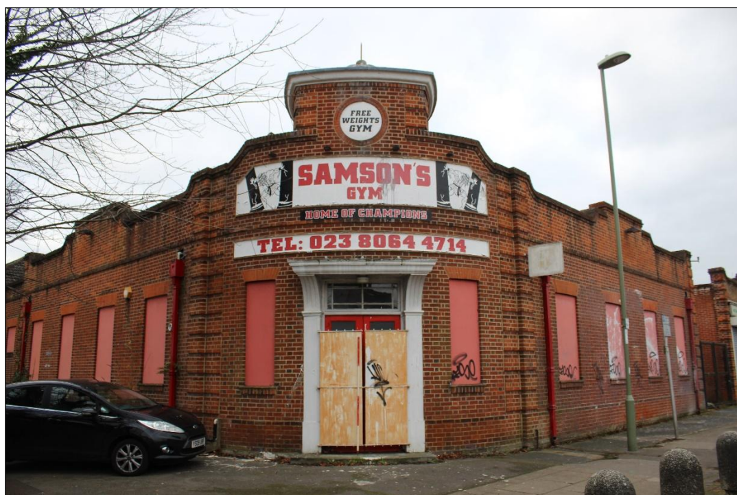
Photo 1 View of the Site from Derby Road (pre-demolition)
