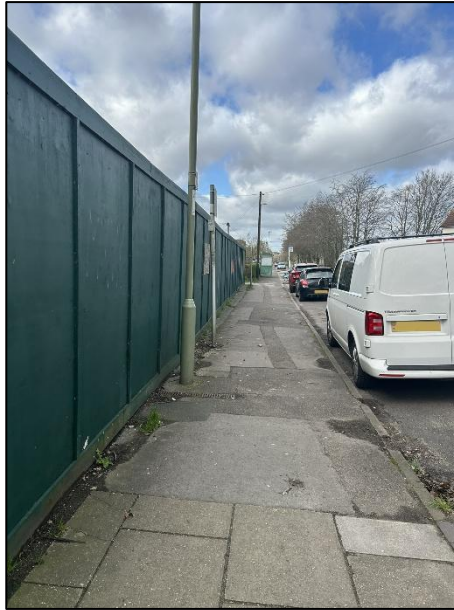
Photograph 2: Site Hoarding on Derby Road
