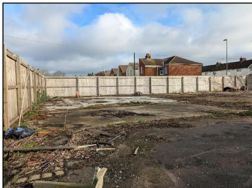
Figure 1: Site comprising developed land, sealed surface
