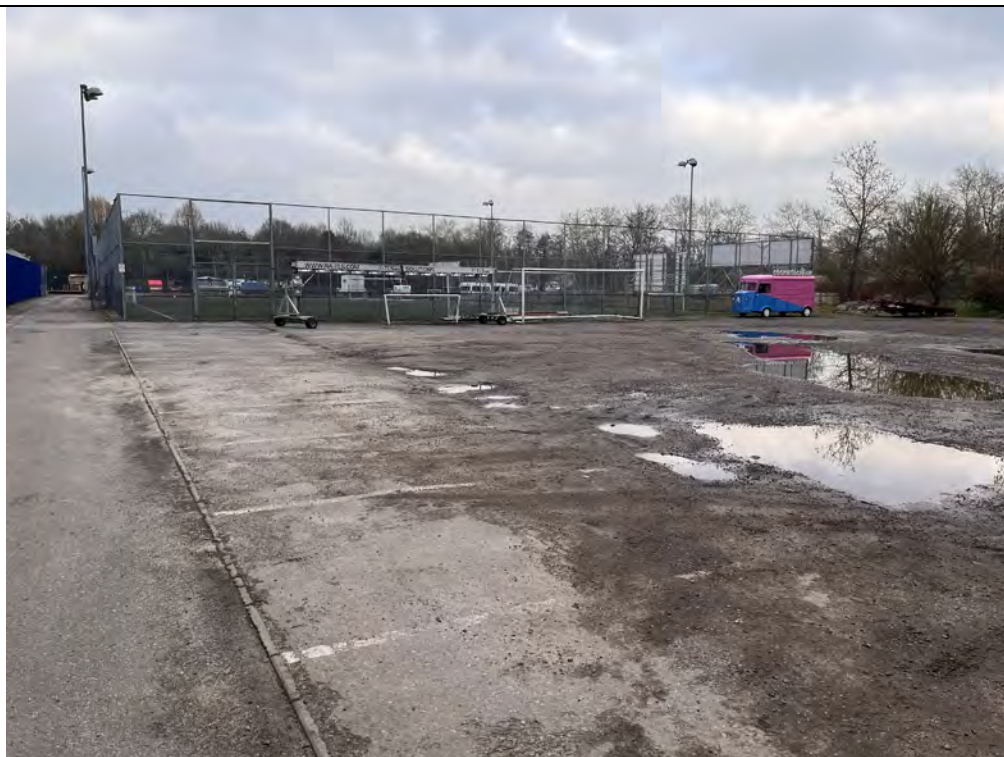
General view of hardstanding on the 9 th March 2026
