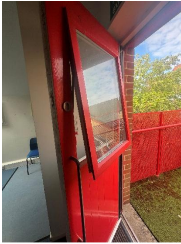
Fig 8. Existing external door to meeting room 26, with openable window
