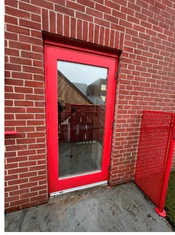
Fig 7. External view of existing fire escape door to external stairs.
