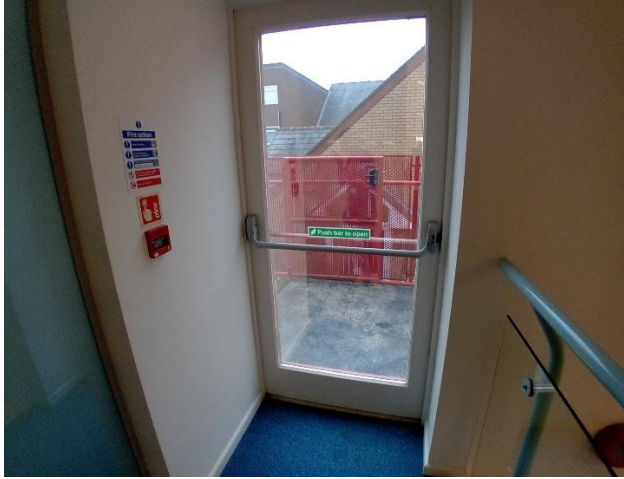
Fig 6. Internal view of existing fire escape door to external stairs
