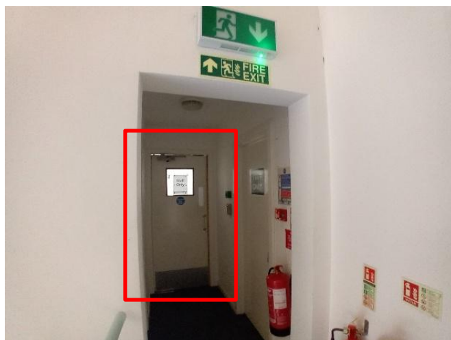
Fig 13. Existing fire door within corridor 14
