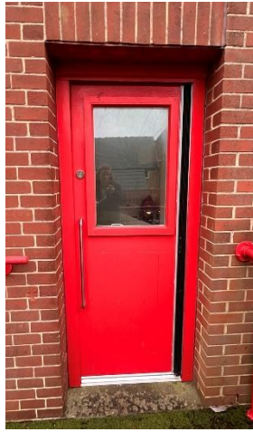
Fig 9. Meeting room door, external
