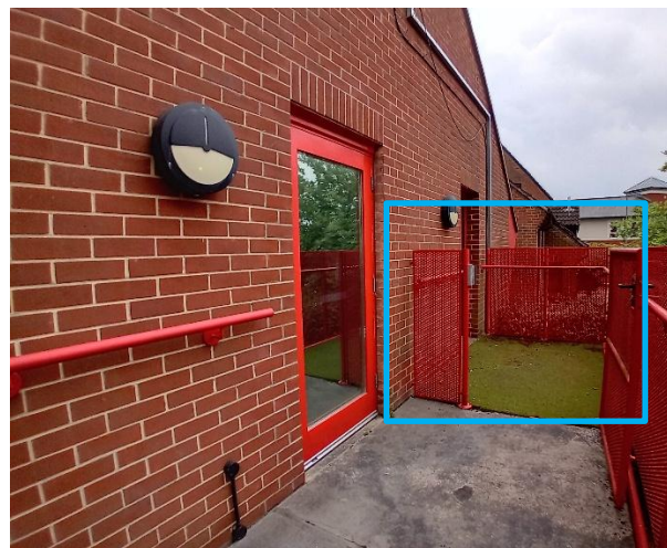
Fig 5. Existing landing at top of external fire escape stairs showing partition with open gate.
