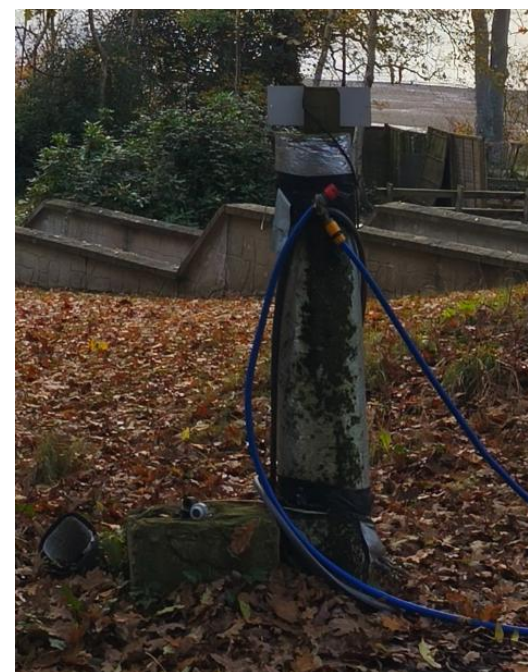
Figure 8: Water access points are onsite at various locations.
