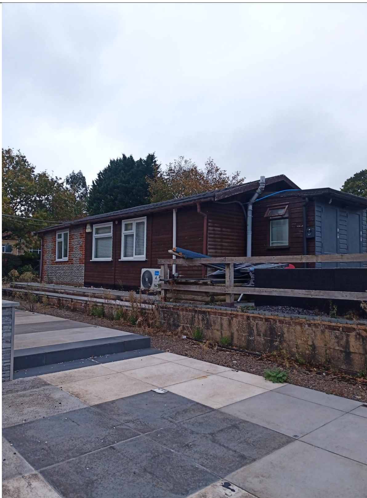
Photo 7: One storey building with pitched roof
