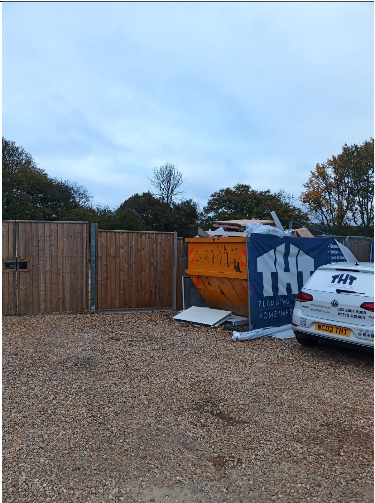
Photo 6: Gravel covered ground was noted and skip onsite
