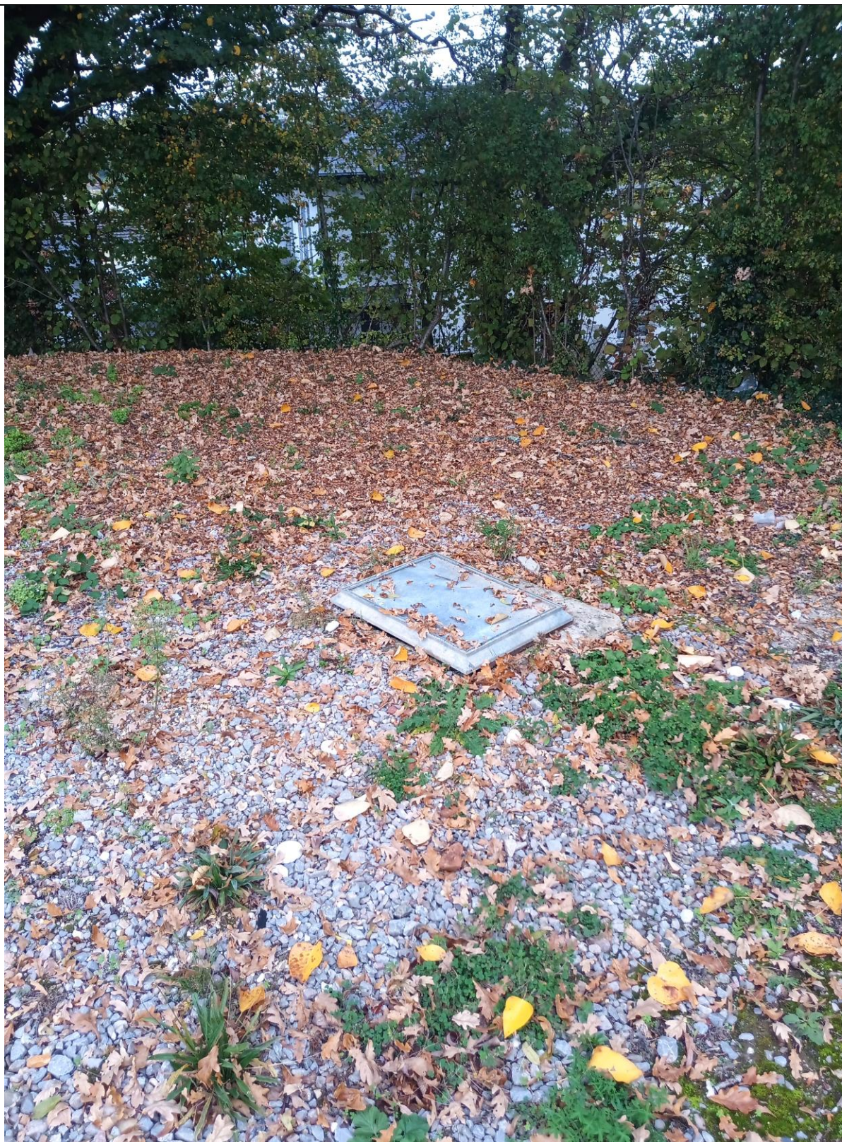
Photo 4: Drainage cover noted onsite
