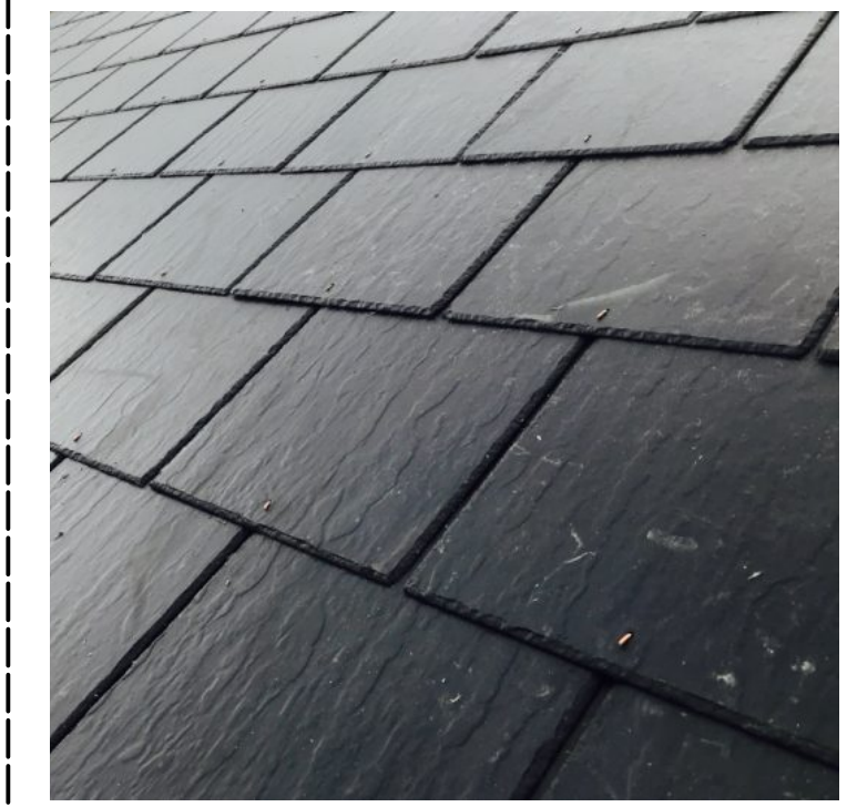
SLATE ROOF TILES
