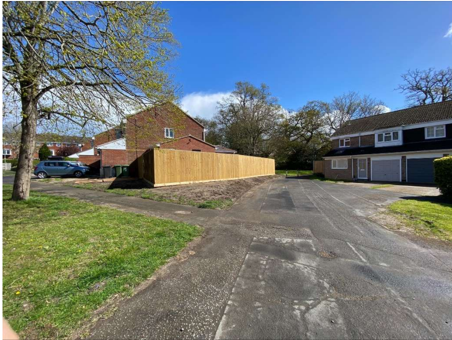
Fig.1 – Photograph showing the erected fence.
