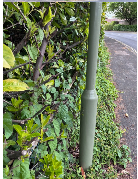
Lampost clearance from existing fence line
