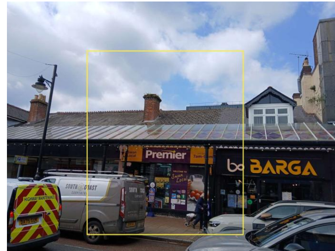
Eastern elevation of B1.
