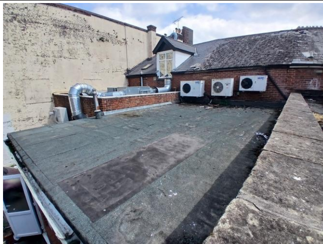
Photo 3: Western flat roof extension.
