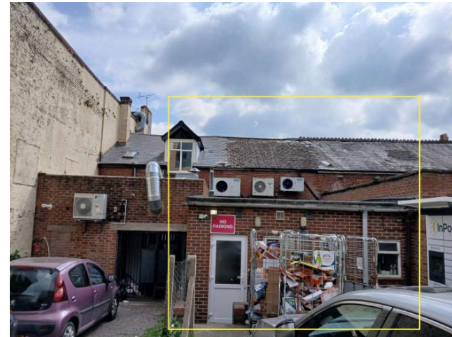
Photo 2: Western elevation of B1.
