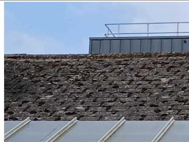
Photo 4: Close up of roof tiles on the eastern elevation.
