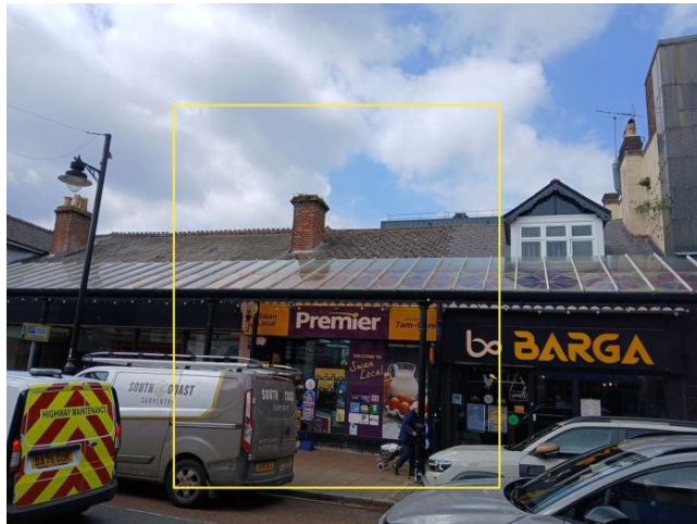
Photo 1: Eastern elevation of B1.
