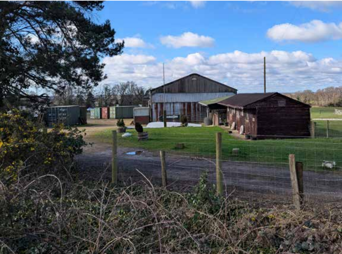
Fig 6.3 - Buildings to be demolished
