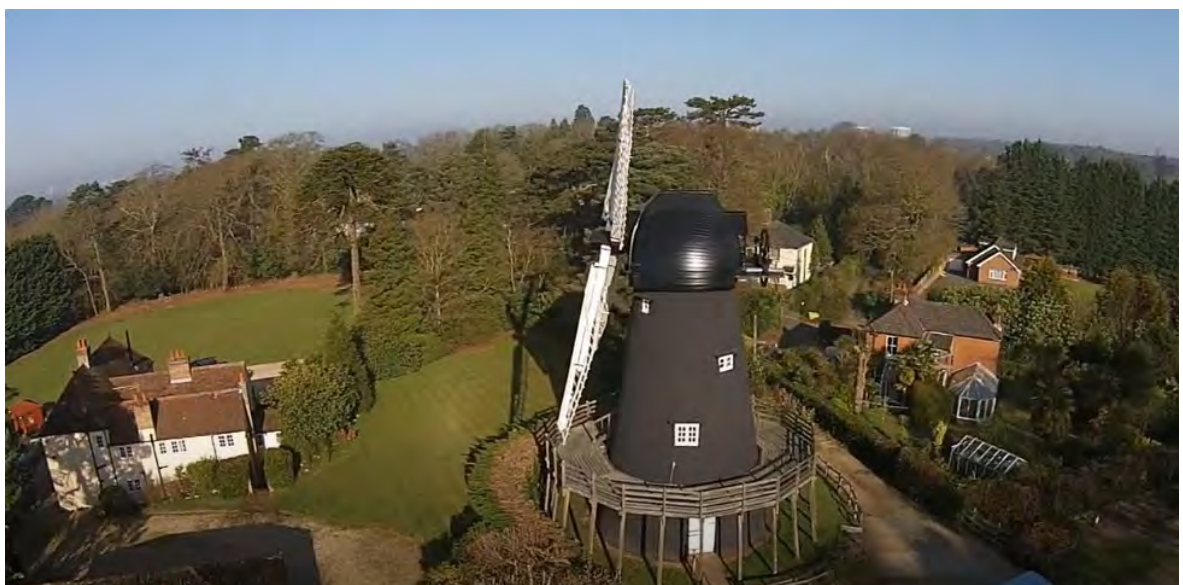
Plate 10: Oblique drone view looking north-west towards the Site over the Bursledon Windmill, showing the extensive tree-cover to the north and west of Bursledon Windmill. The curved horizon is a product of the fish-eye technology. The Windmill sits on a relatively flat plateau
