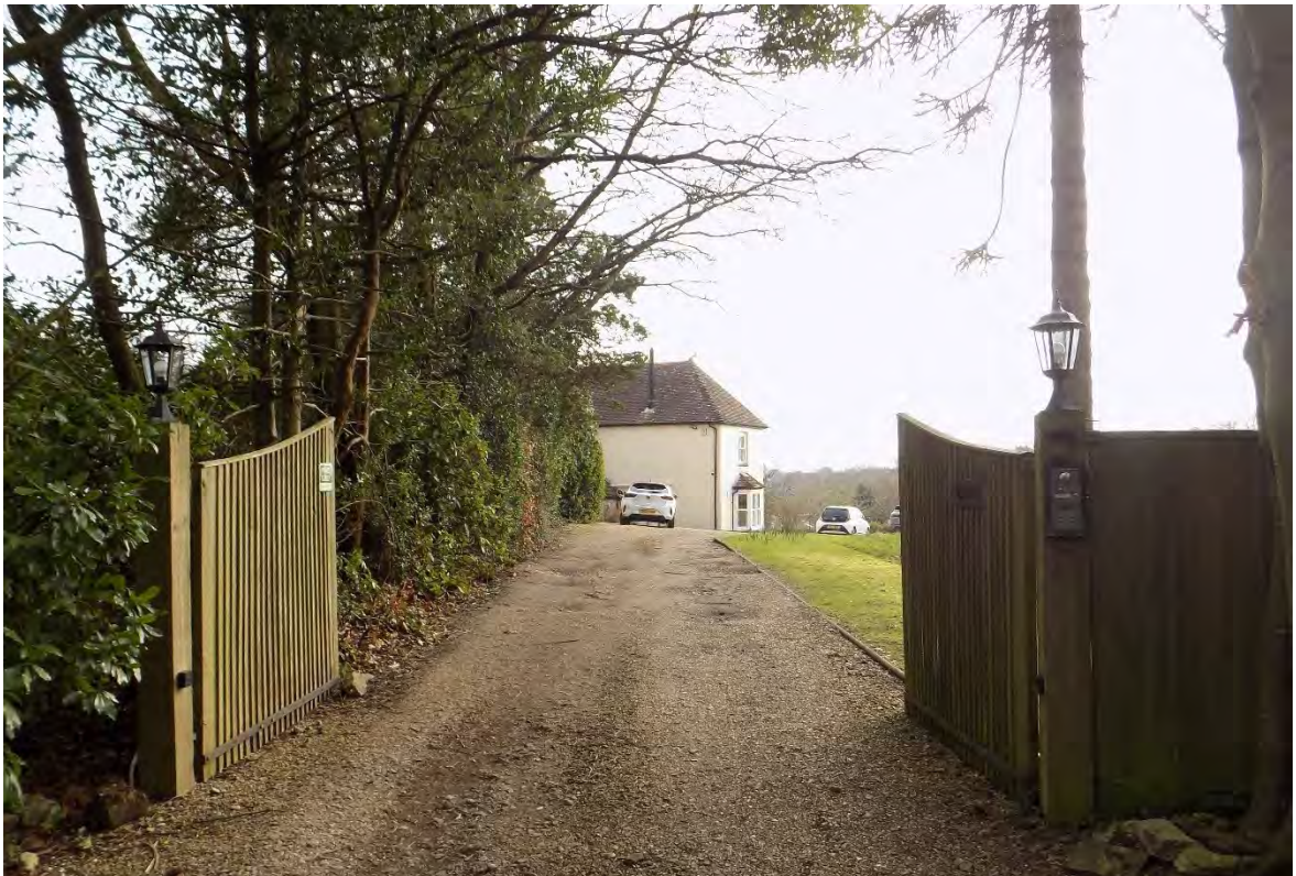
Plate 6: View of the non-designated Mill House at Bursledon Windmill, as seen looking south from, Windmill Lane. The house is now a private residence and is separated from the windmill with a belt of trees
