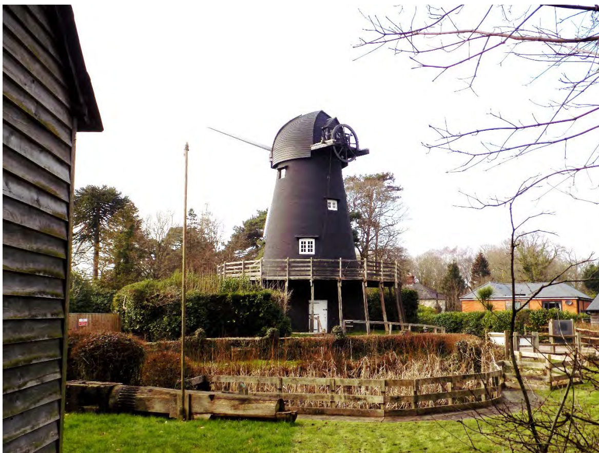
Plate 4: View of the Grade II* Bursledon Windmill, looking north-west towards the Site
