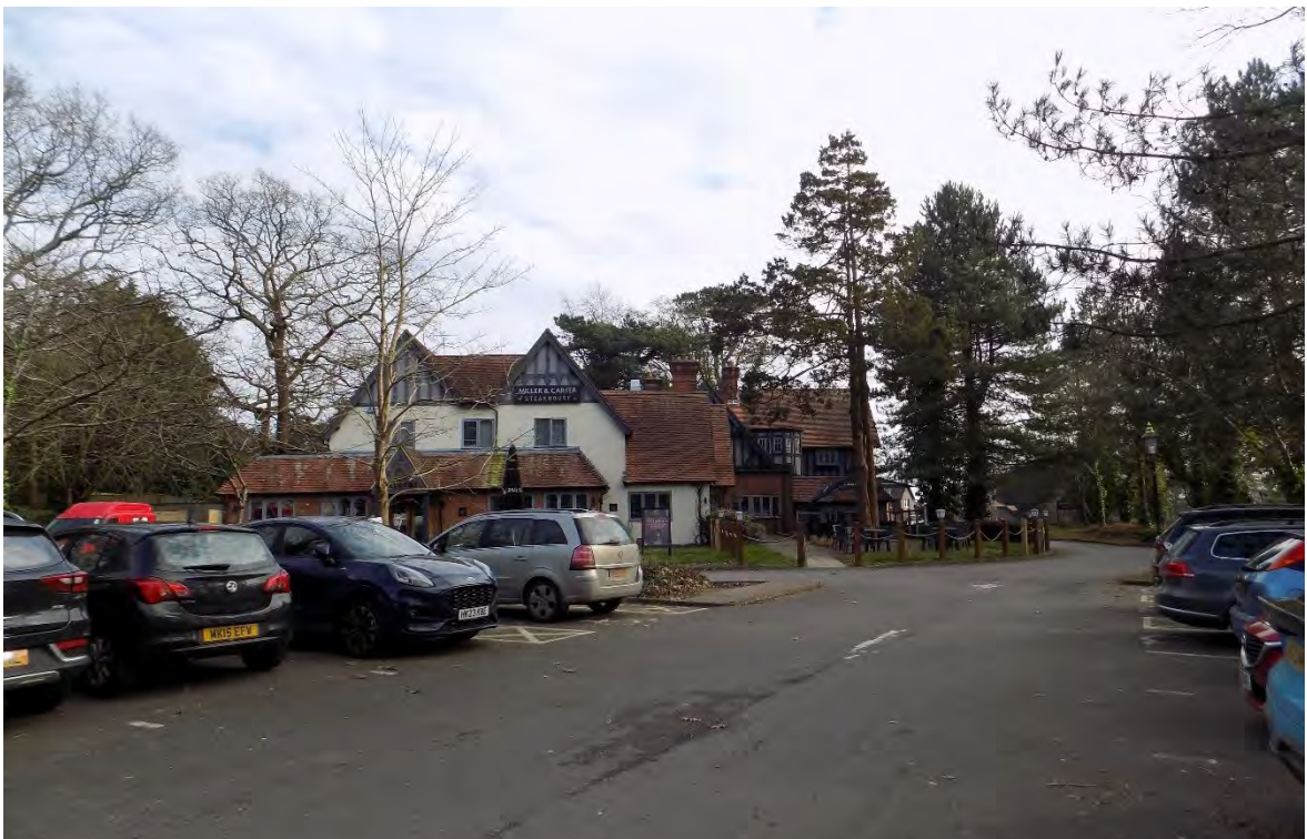
Plate 8: View of the large modern rear extensions to the locally-listed Miller & Carter steakhouse (formerly Evysley), looking south-east from its extensive car-parking
