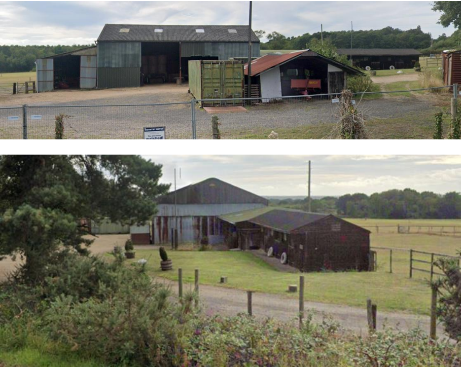
Figure 6: Examples of existing buildings on site
