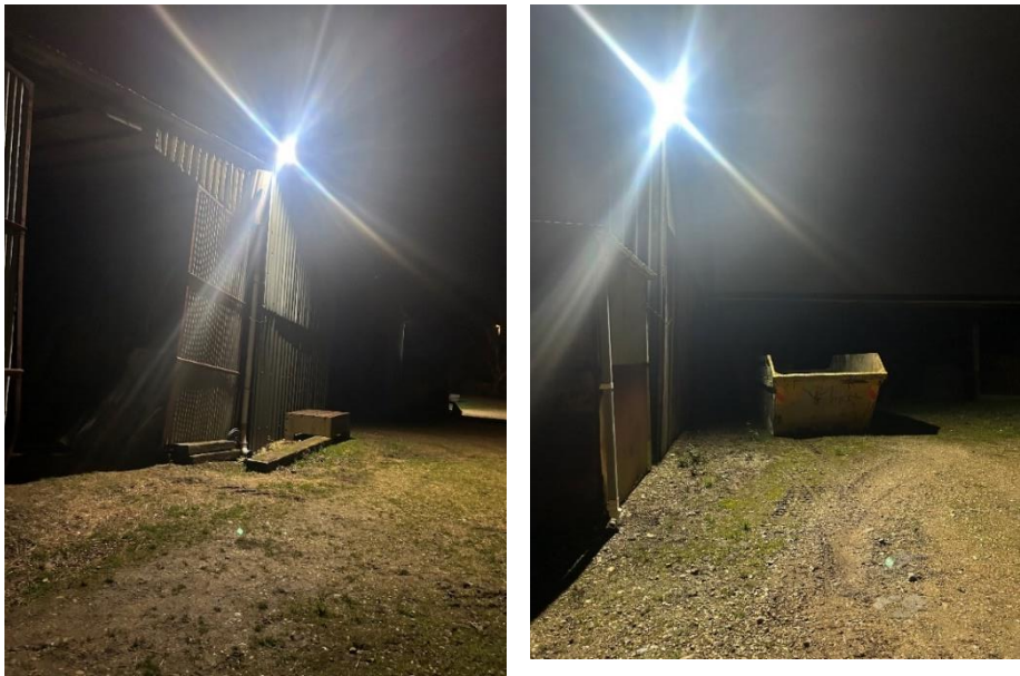
Figure 6. 5: Point 28 & 29 – Existing Lighting. Taken during a night survey on 13 February 2025
