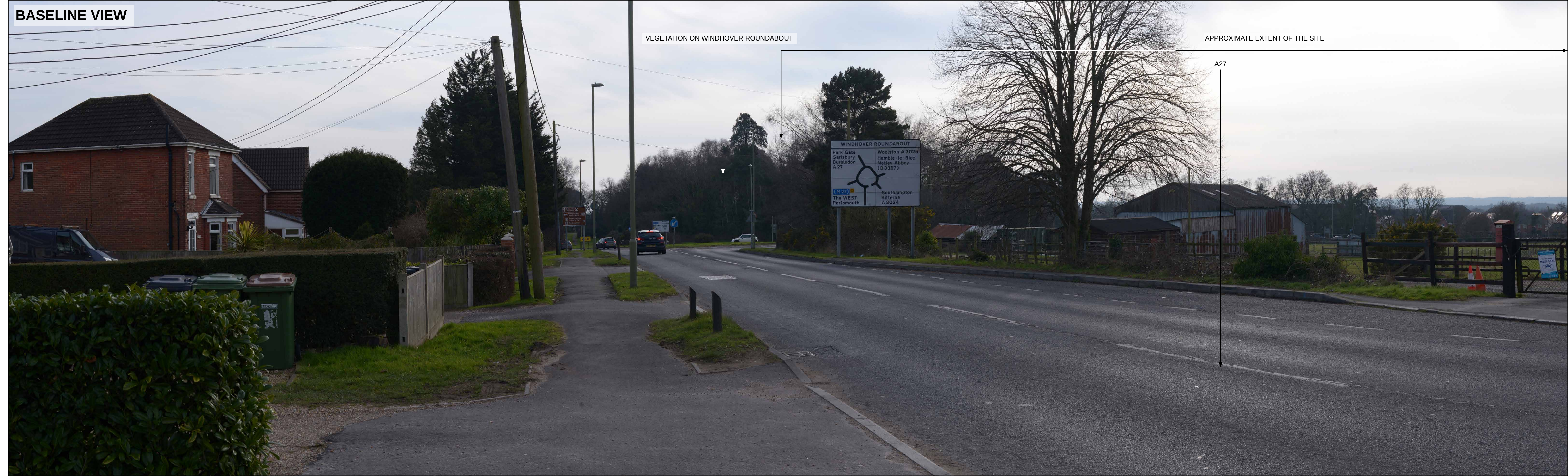
VIEWPOINT:8 VIEW FROM A27/ WEST END ROAD, LOOKING SOUTH TOWARDS THE SITE.
