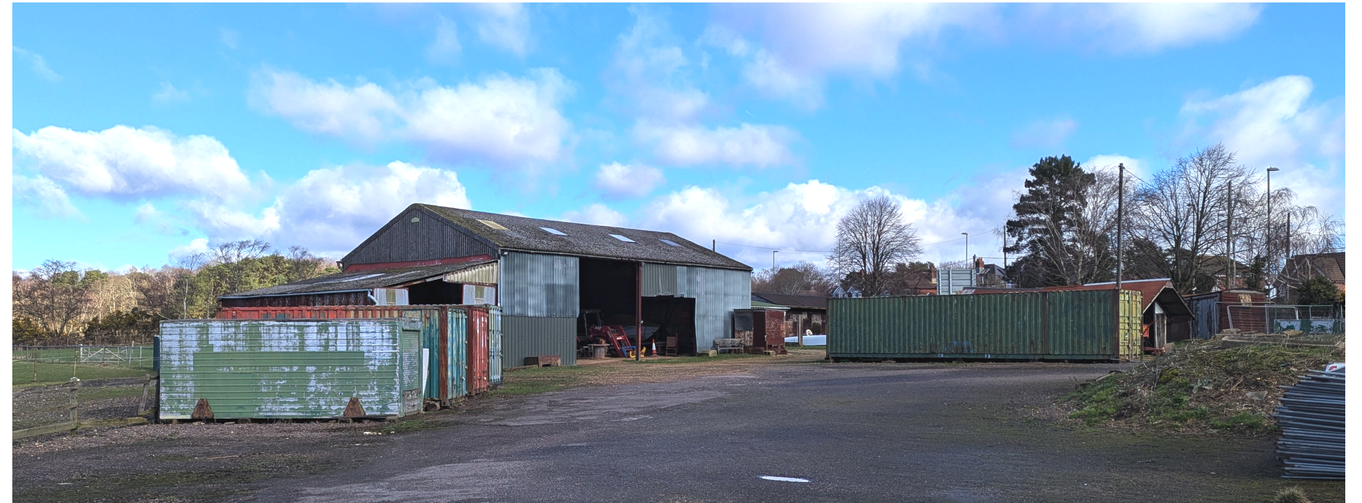
View of buildings to be demolished from the south
