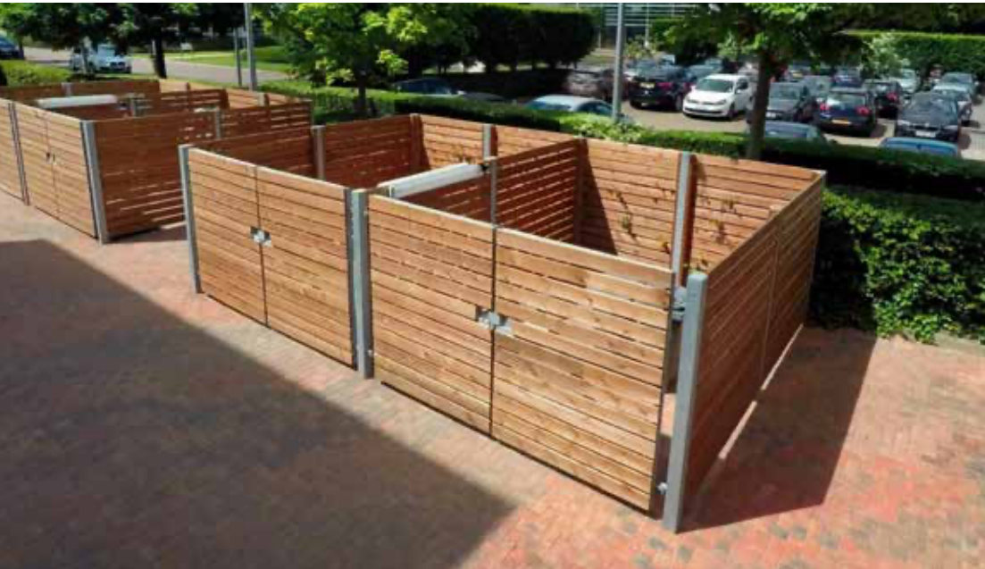
Figure 7.13 Typical commercial bin store enclosure
