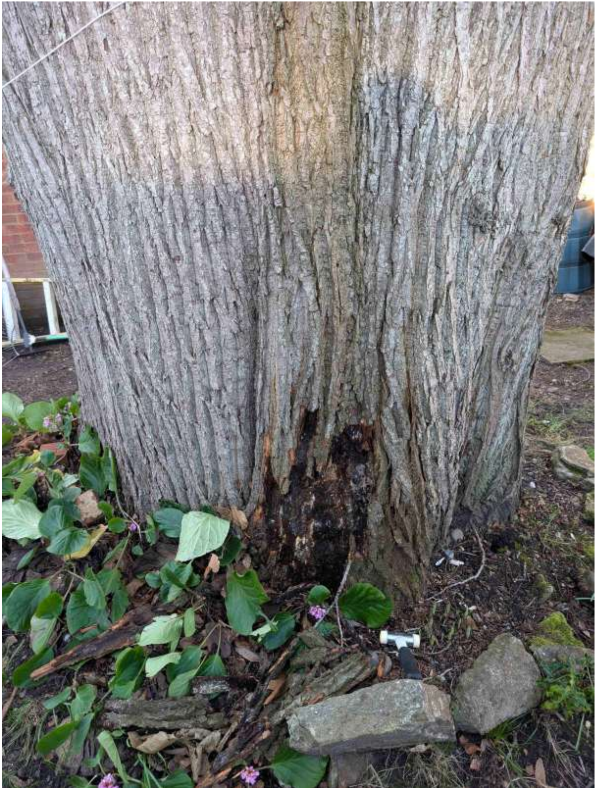
Figure 1: East side of base, area of decay
