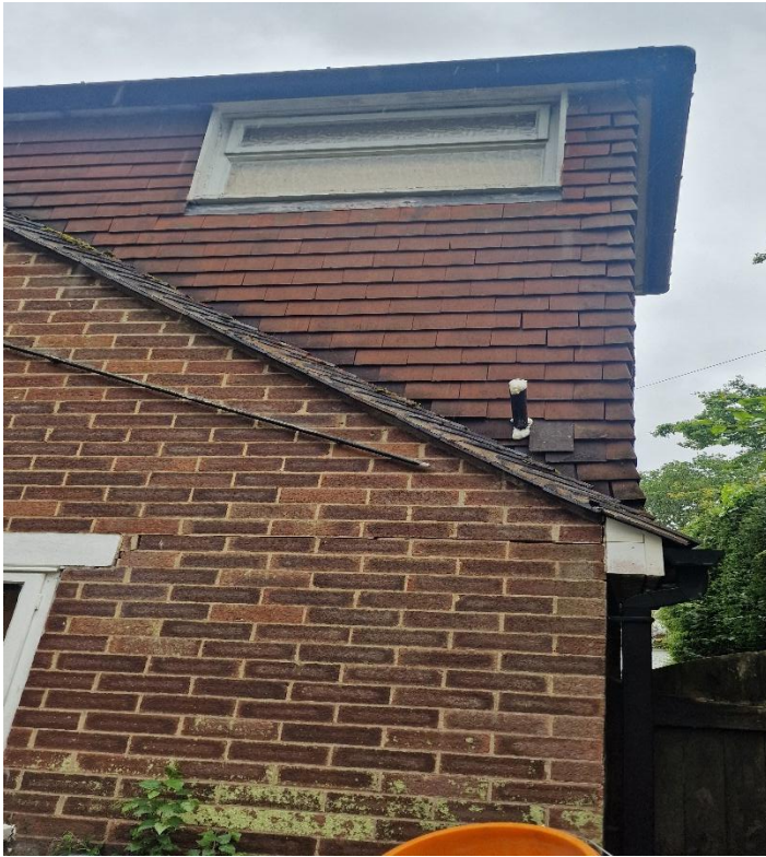
Picture 3: Showing the tile hanging on the western dormer
