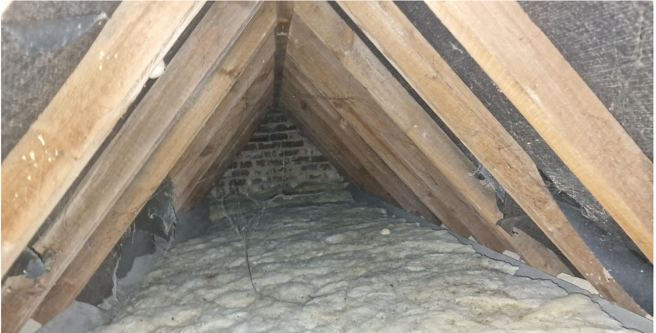
Picture 7: Showing the roof void
