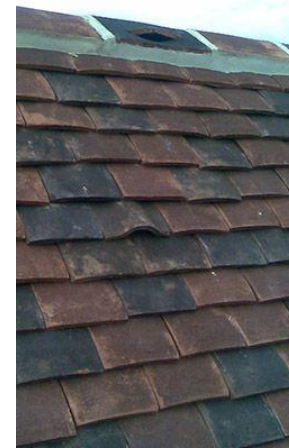
Roof access tiles with bitumen felt underneath
