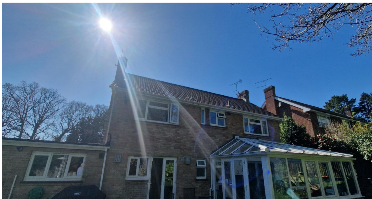
Picture 3: Showing rear elevation
