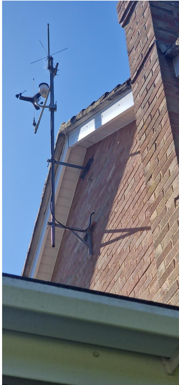
Picture 5: Showing the eaves at the eastern end
