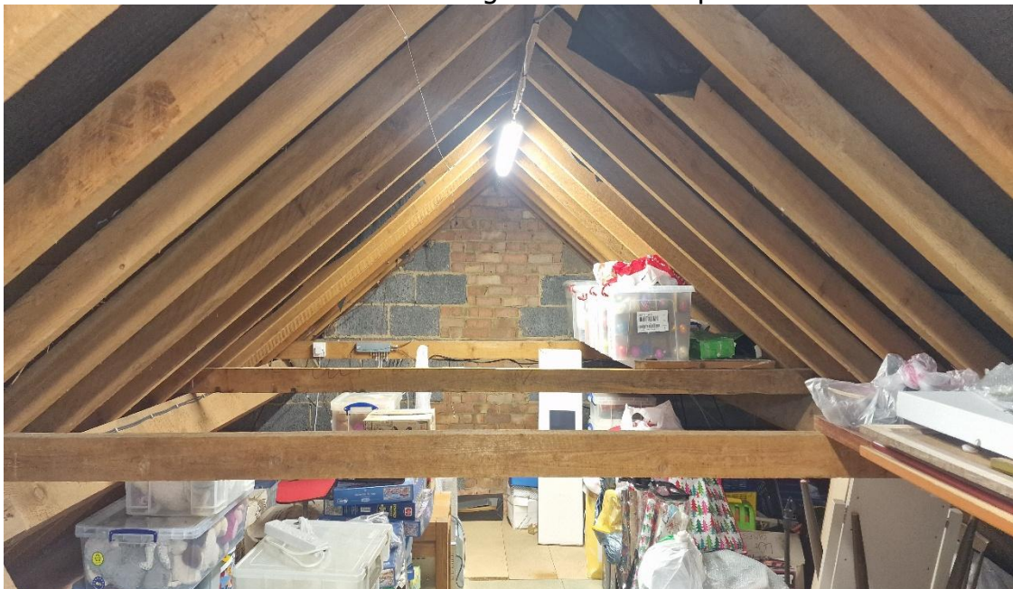
Picture 10: Showing the internal structure of the roof void
