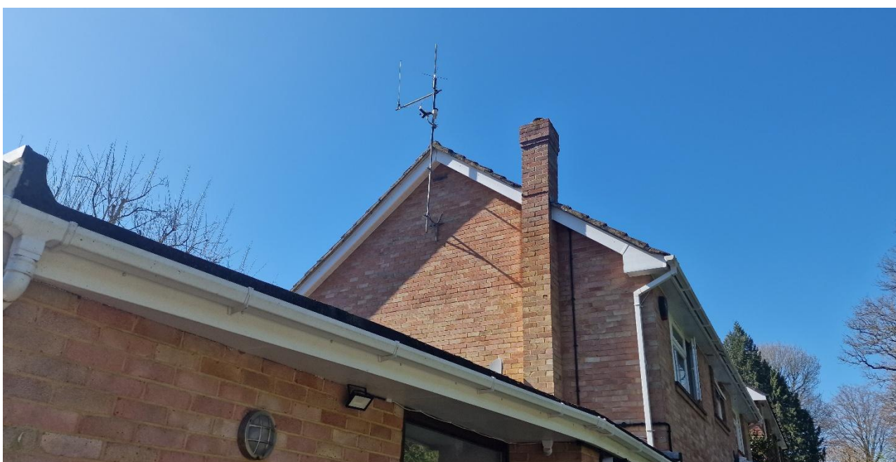
Picture 4: Showing the rear elevation
