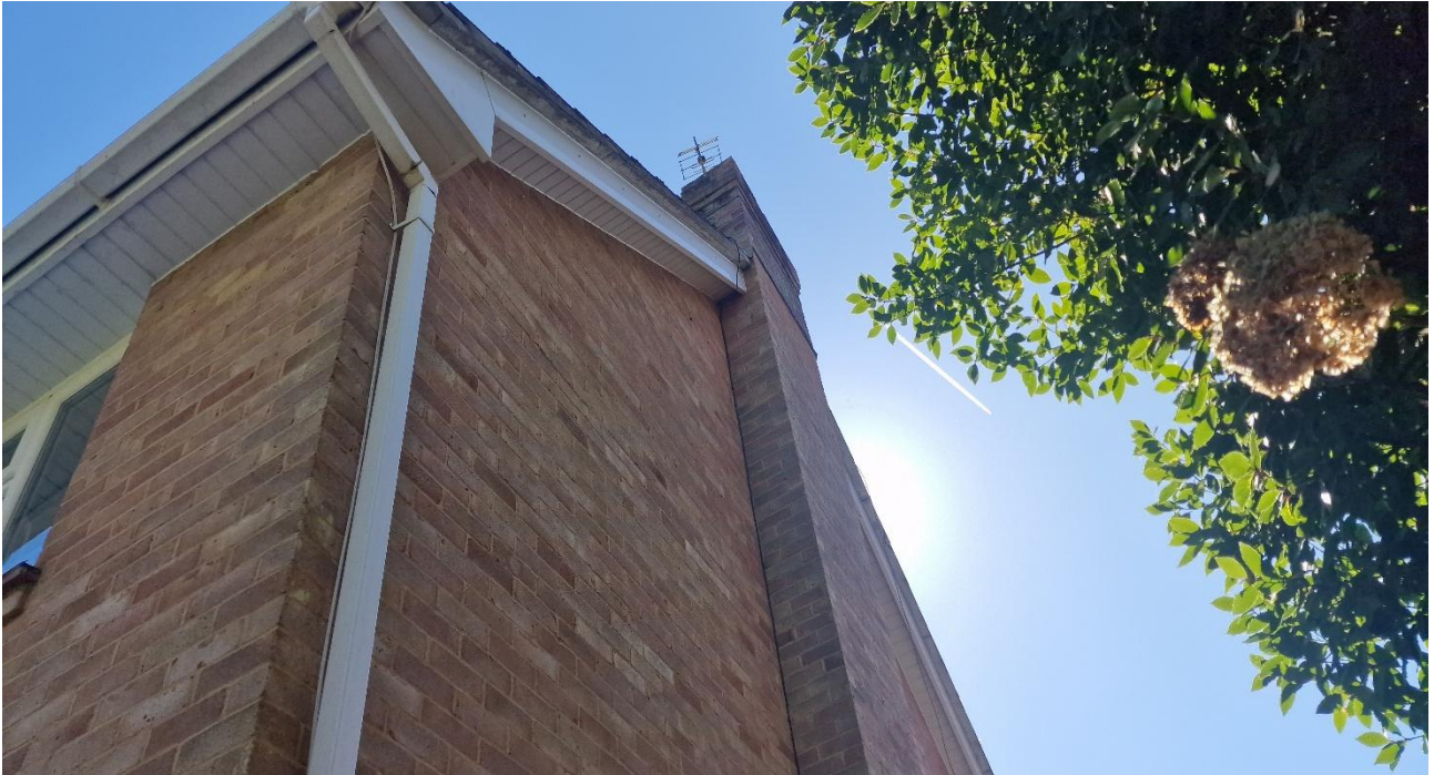
Picture 6: Showing the gable wall of the western elevation
