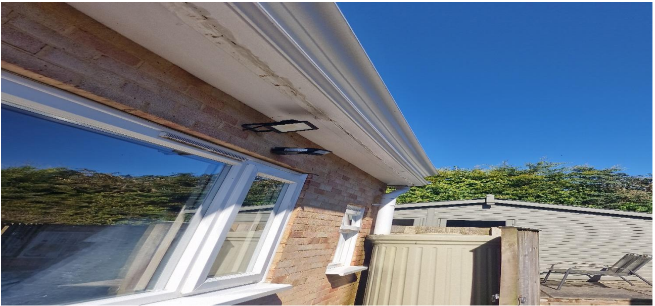
Picture 8: Showing the eaves of the garage
