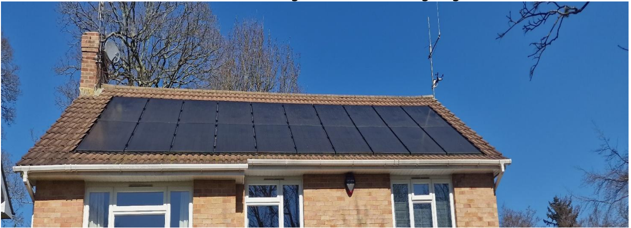
Picture 9: Showing the flush solar panels
