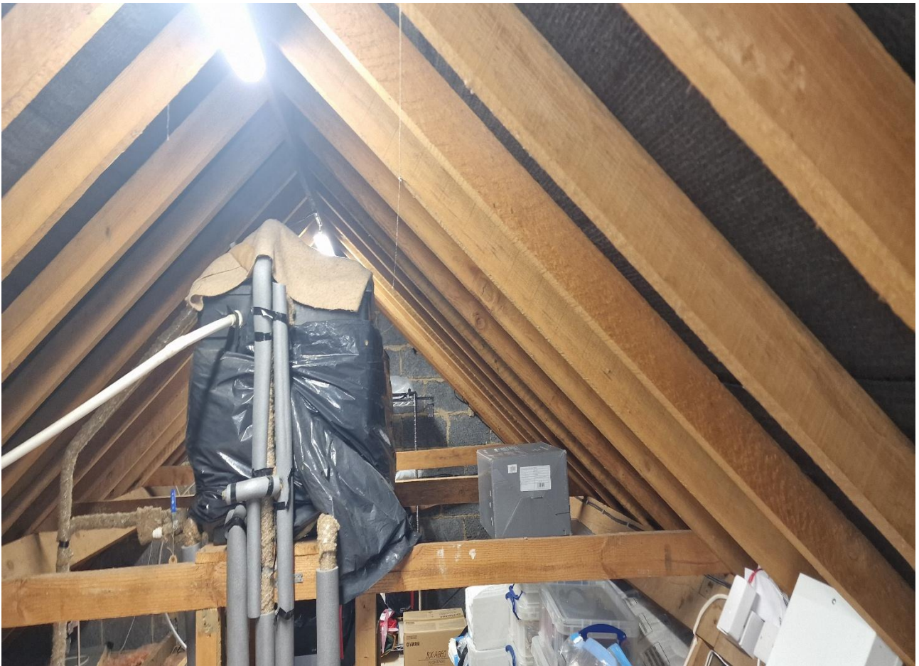
Picture 11: Showing the internal roof void
