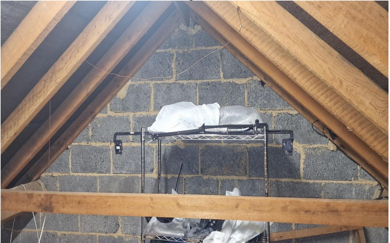
Picture 12: Showing the internal roof void
