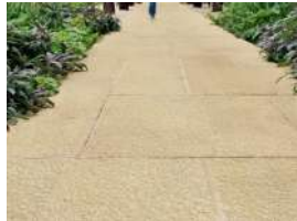
Paving slabs in buff finish to patios and communal terrace
