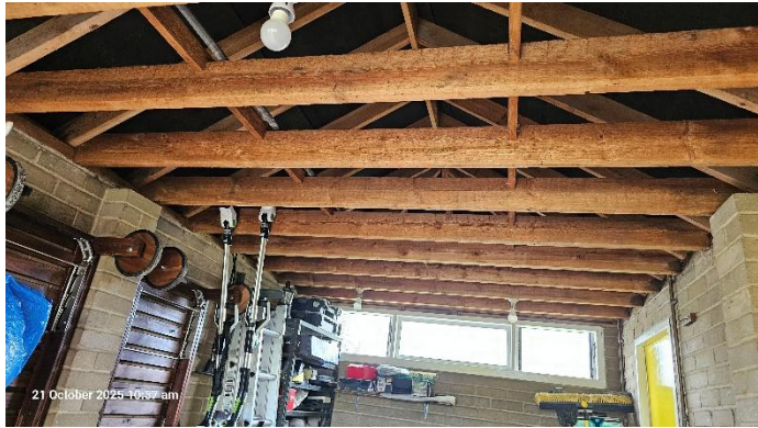
Photo 7: Internal view of garage.
