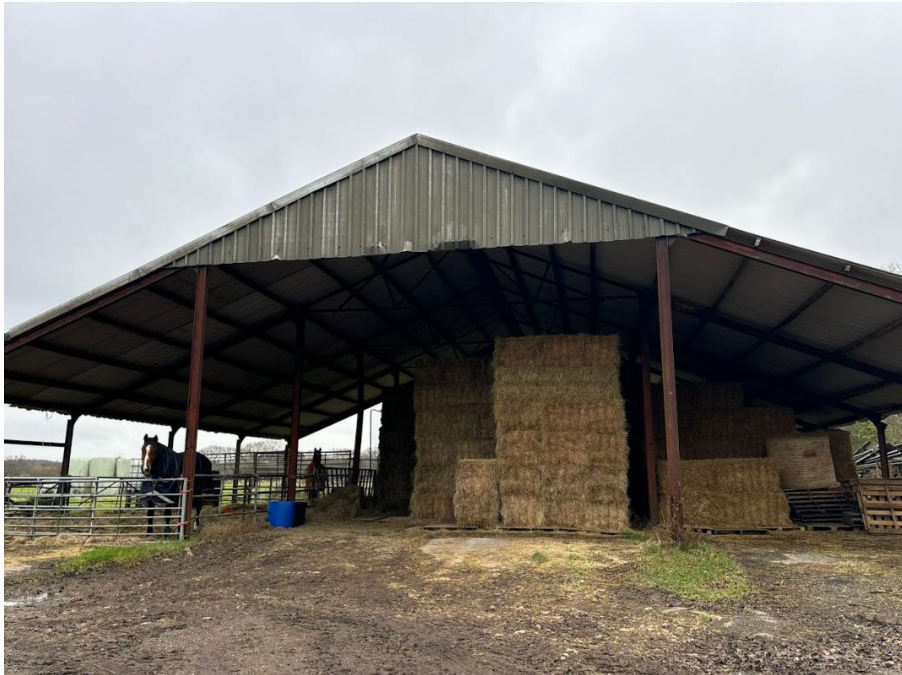
Figure 6. View of the barn on site (taken December 2024).
