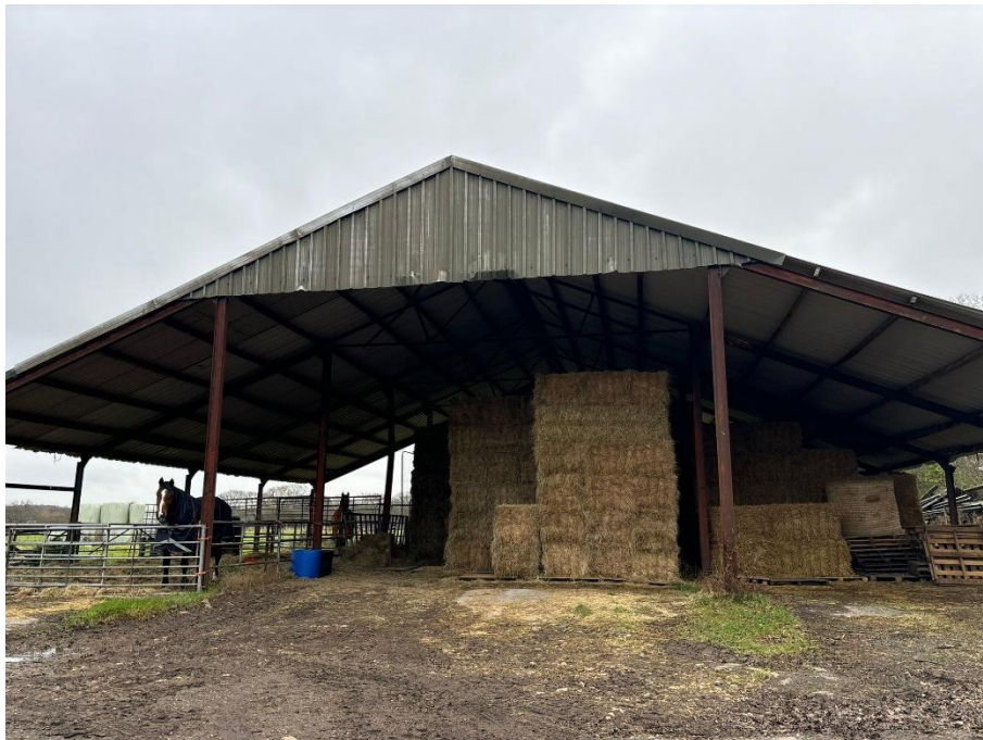
Figure 5. View of the hardstanding in front of the barn at the south of the site, looking east (taken December 2024).
