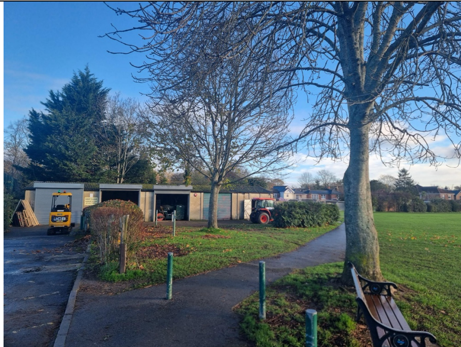
Front showing roller doors
