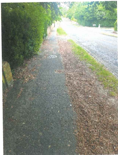
View of pavement heading down Hiltingbury Road, from Oakwood Road towards Oakwood Close
