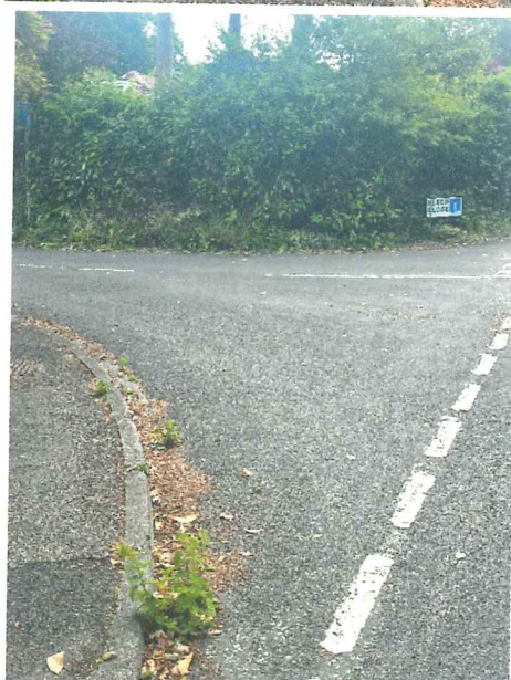
Beech Close – will need to be crossed and no dropped kerb
