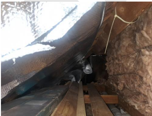
Figure 5. Internal view of eaves voids.
