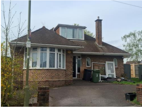
Figure 1. External image of eastern elevation.
