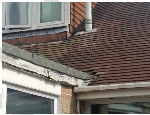
Figure 4. Raised tiles near to flat roof extensions and gaps in fascias.
