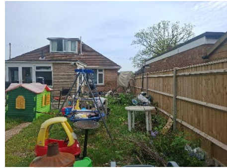
Figure 2. External image of western elevation.
