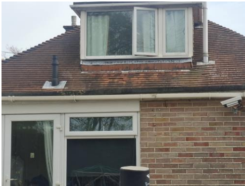
Figure 3. Dormer on western elevation.
