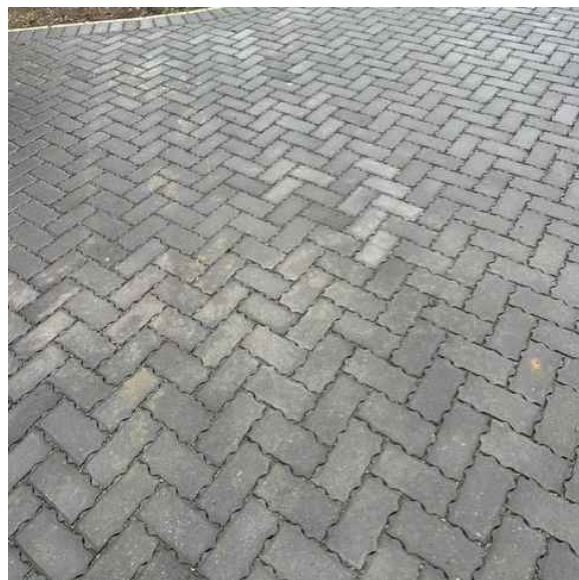
B Light grey permeable block paving
