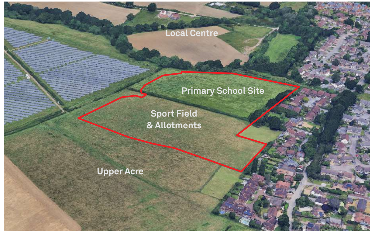
Aerial view from south-east
