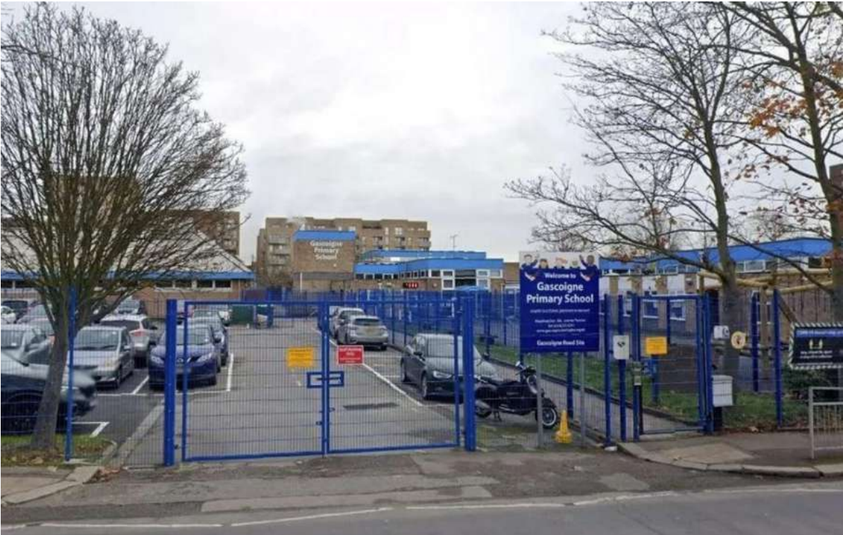
Typical school set defensively behind fences and dominated by parking to the front
